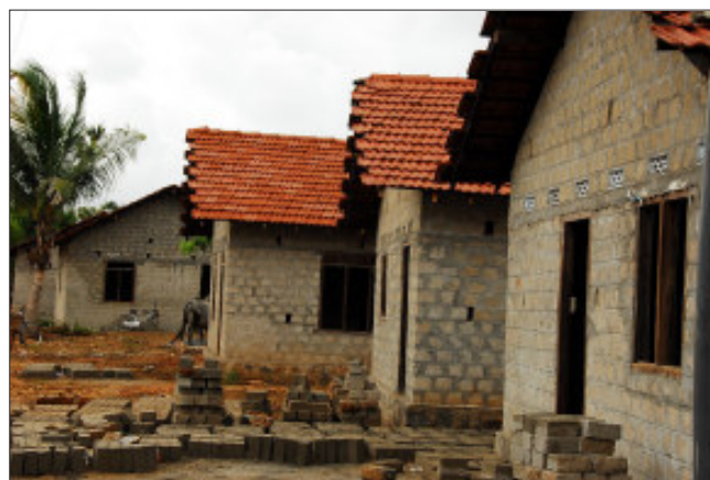
Houses being constructed through an American Red Cross owner-driven housing initiative in Sri Lanka.
