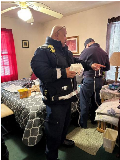
College Park, Georgia Fire Department members install a bed shaker smoke alarm.
