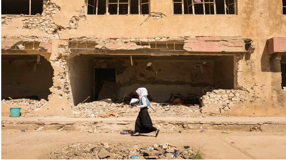
Photo Credit: Robin Hammond, ICRC. Al-Raja secondary school for girls, Anbar, Ramadi, Iraq. It was in large destroyed during the last conflict, 2017
