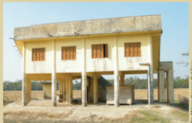
Cyclone-resistant shelters like this one have saved countless lives.
